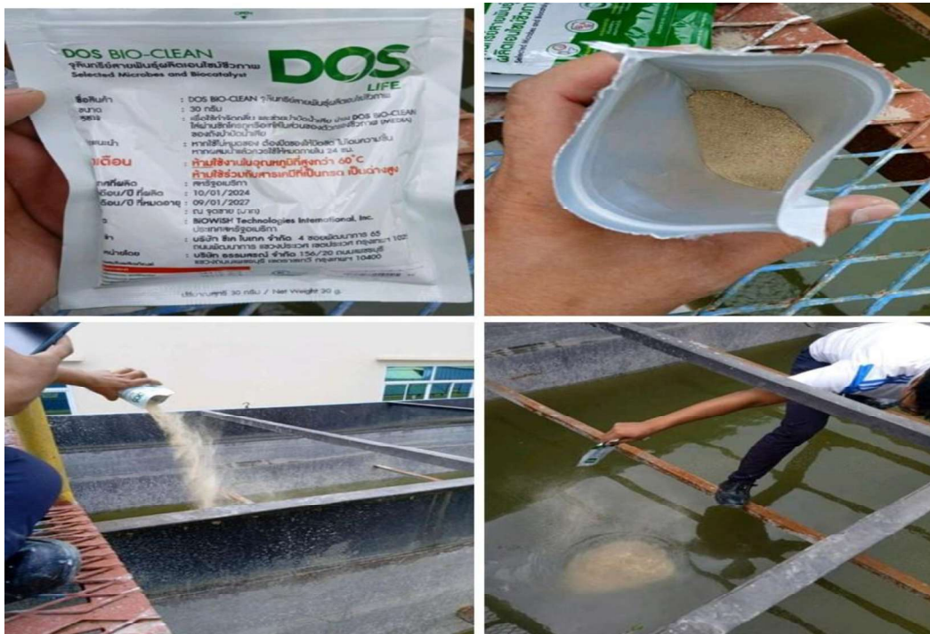
Figure 3-14 Microorganism used in wastewater treatment plant and photo of adding to treatment plant
