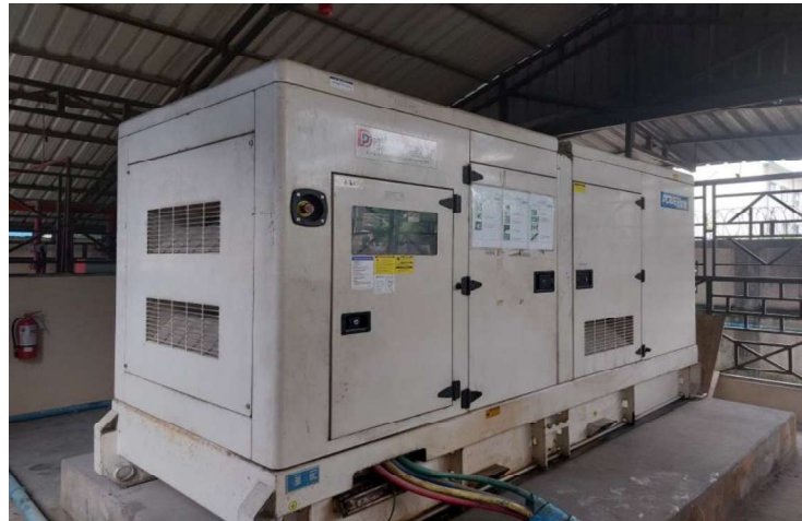
Figure 3-12 photograph of generator, 250 KVA
