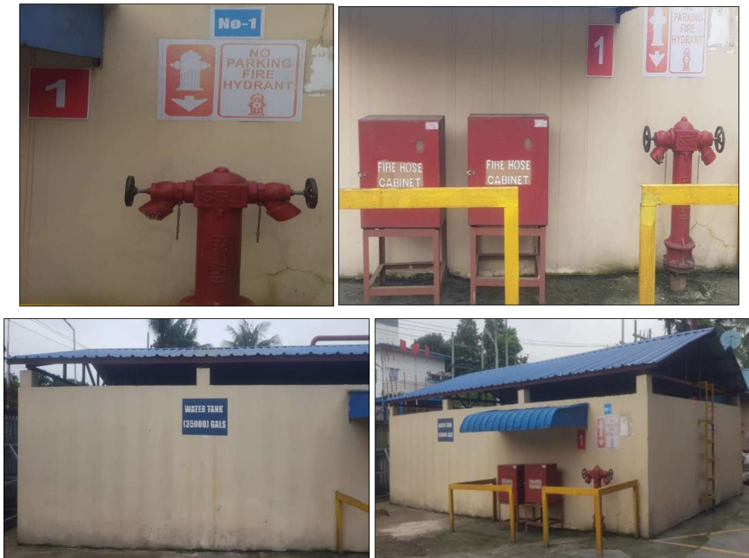
Figure 7-21 Fire Hydrants and Water Tank for Firefighting
